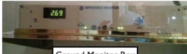
Ground Monitor Box
