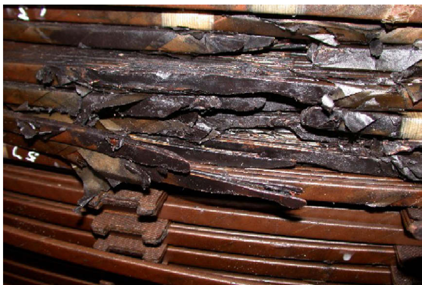
Fig. 4. Failure in a large South African generator transformer three weeks after the Halloween storm of October 2003. The disruption of the winding and insulation by the arcing fault at the time of final failure is clear. The arcing fault also destroys evidence that might lead to a better understanding of the progression of damage after initiation by the geomagnetic current event. (For interpretation of the references to colour in this figure, the reader is referred to the web version of this paper.)
