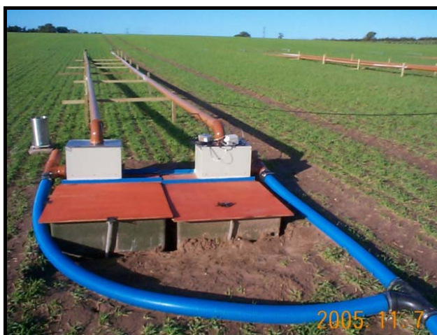
Plate 1b. Piping diverted runoff downslope into the tipping-bucket sample splitters, which directed a representative subsample of runoff into covered storage tanks. The remaining runoff was directed to waste.
